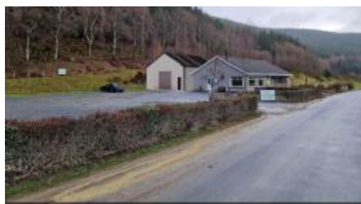
View from north approach
